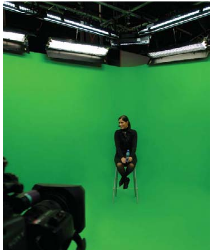
HD virtual studio with Image 85 DMX fixtures and 4ft Double systems
